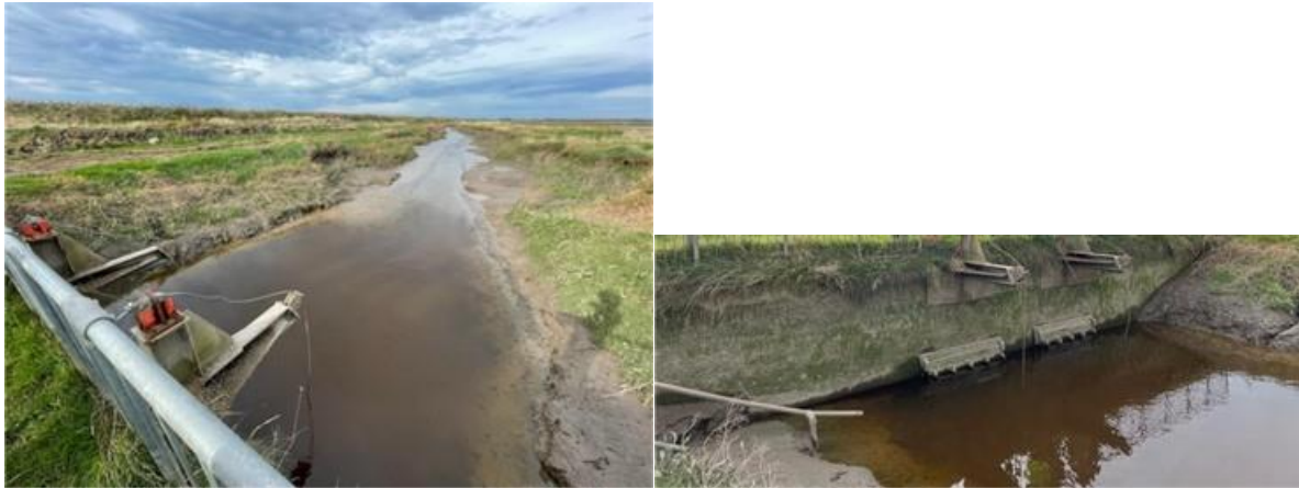
Figure 5.17 Outflow at Hundred End Gutter silted up causing water to pool
