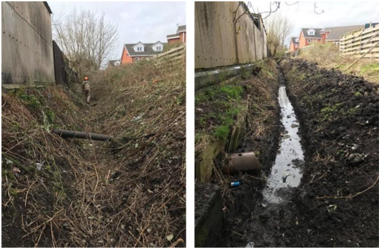
Figure 6.8 Watercourse 16 culvert overflow ditch, during (left) and following (right) clearance
