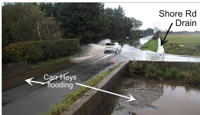
Figure 5.10 Overflow of the Carr Heys draining off the road into Dunkirk Dib
