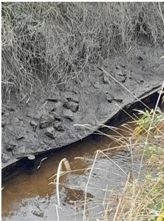
Figure 5.15 Revetment boards pushed into flow
