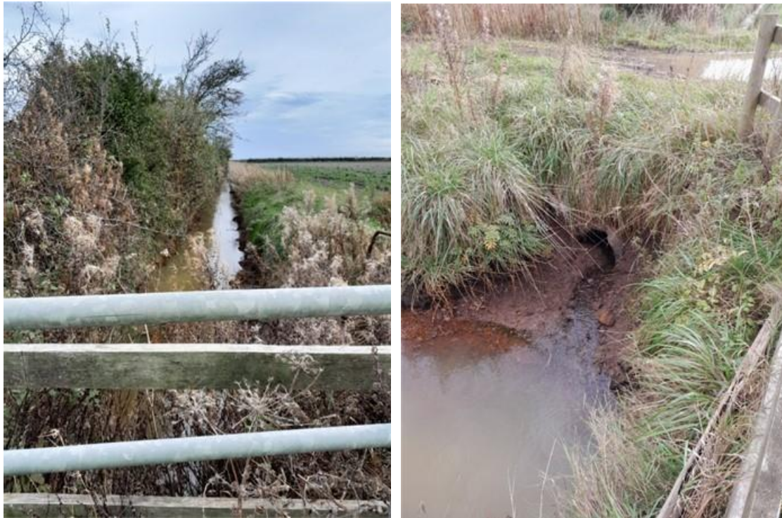
Figure 5.13 Poorly maintained culvert on New Bank Drain
