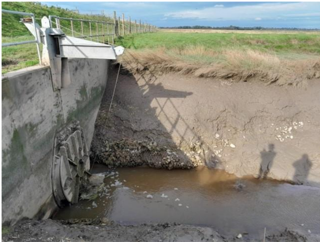
Figure 5.16 Tidal gate at the combined outflow of Centre Drain and New Bank Drain
