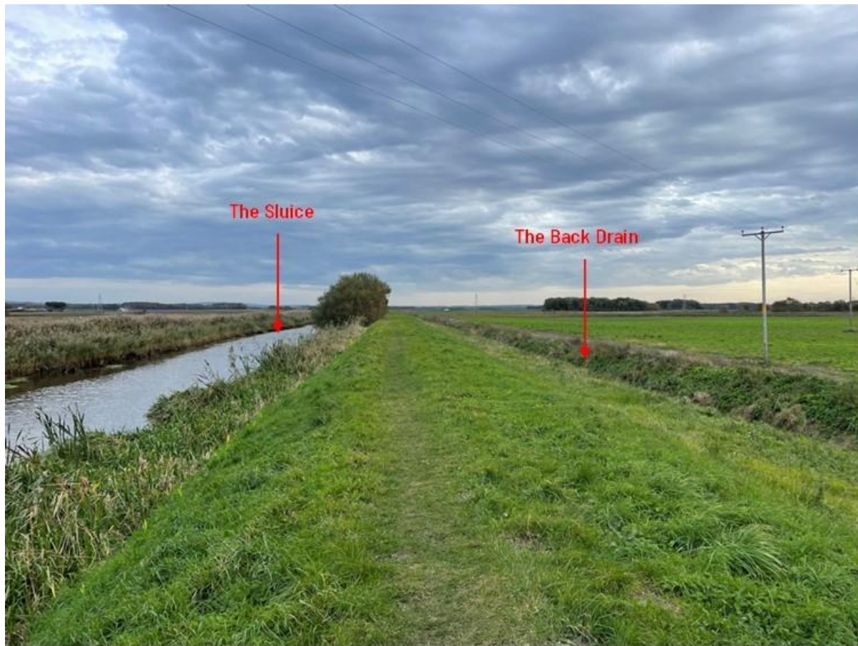
Figure 6.2 The Sluice (high level) and Back Drain (low level)
