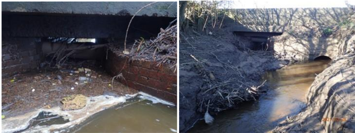
Figure 5.9 Carr Heys culvert under Shore Road – partially blocked by silt and debris
