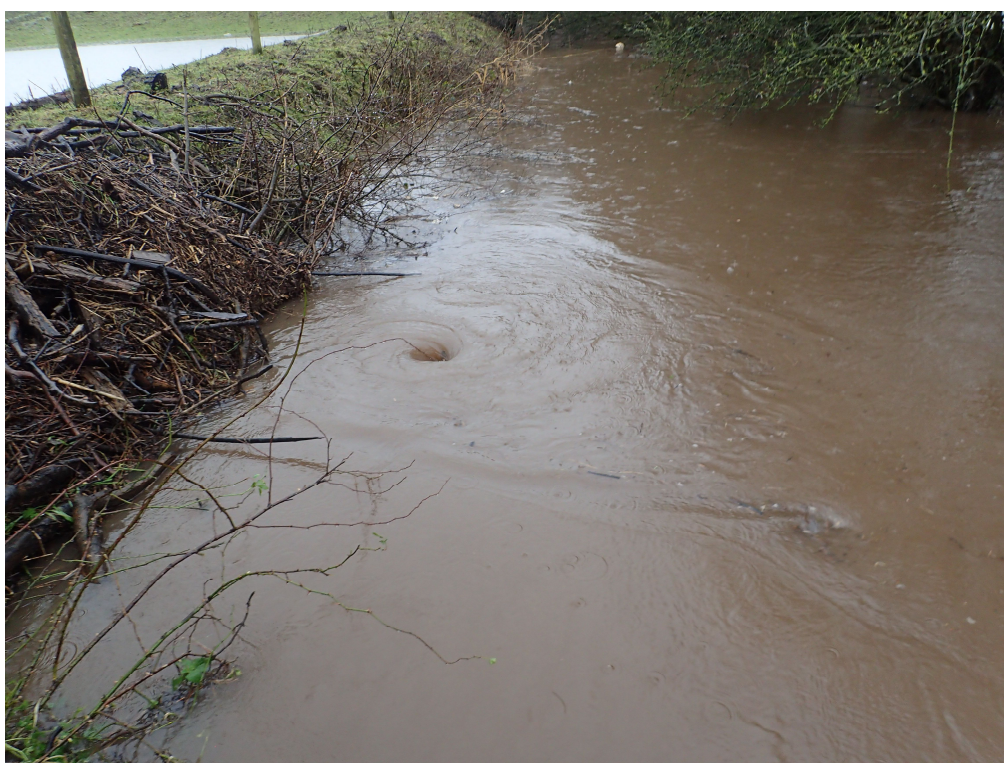
CHW whirlpool possible water sucking through pipe culvert 19.01.2021.
